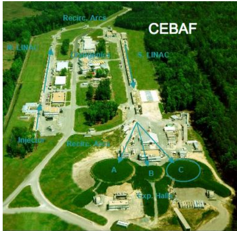
Figure 5. Aerial picture of CEBAF
