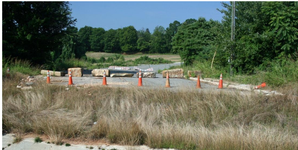
Figure 4.3. Greyhound Court Bridge, southwest approach. View from end of span B.
