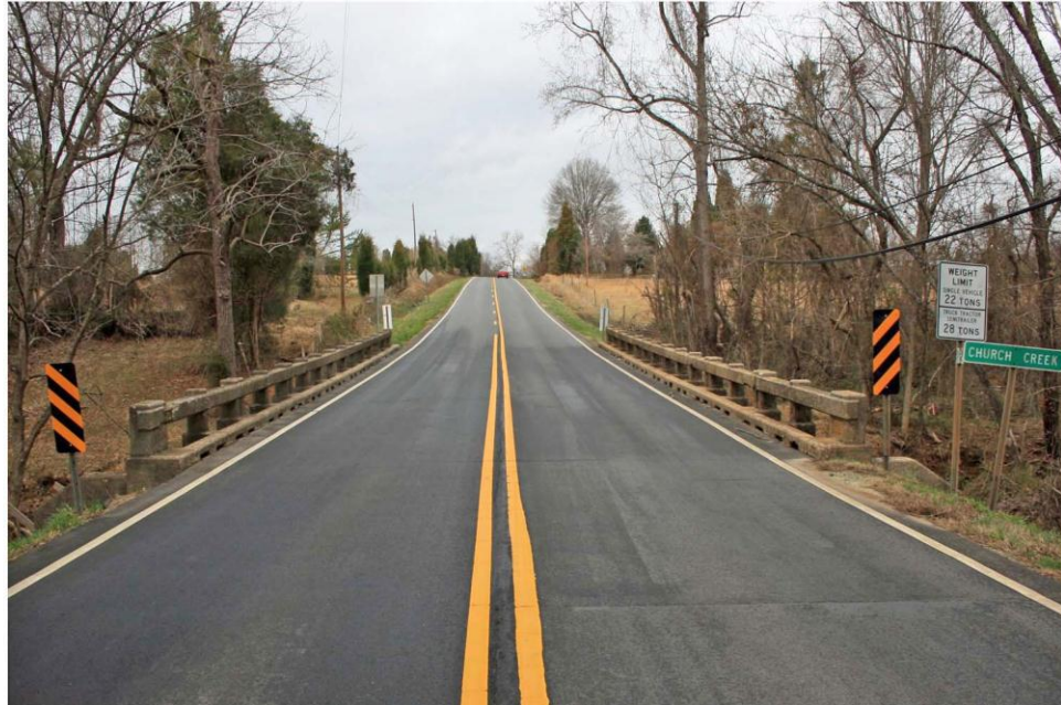
Figure 1.2. Church Creek Bridge looking east.
