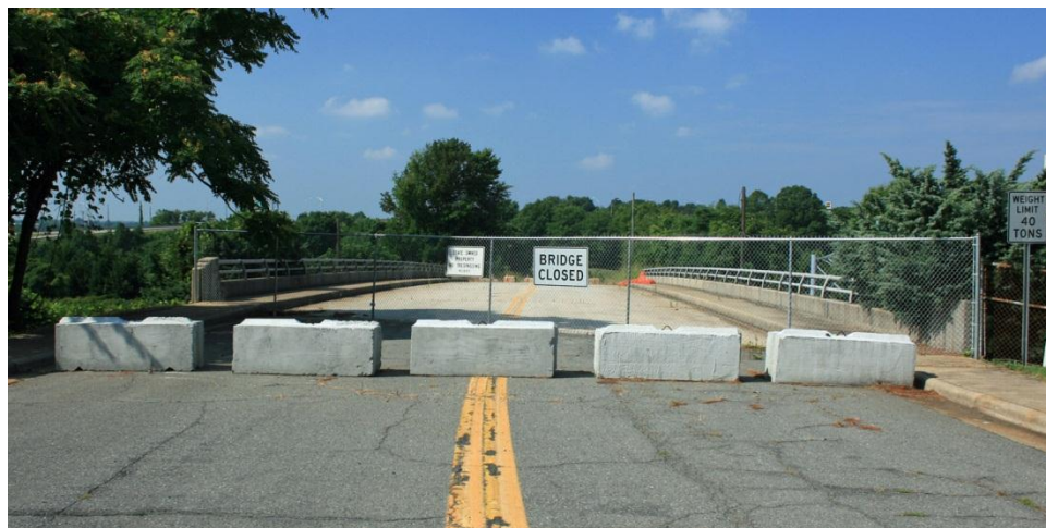
Figure 4.4. Greyhound Court Bridge, northeast approach.
