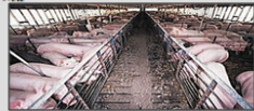
Figure 1. Indoor housing management operations, shown as a group of confinement operations. As you can see in the photo, there is a wide abundance of space for the piglets and an air flow that helps the circulation in the indoor air, intake and organic matter.
