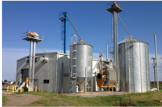
Figure 8. Crop Processing Facility.
