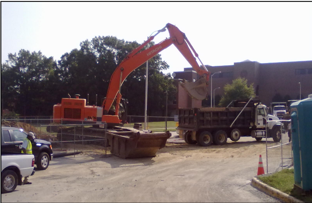
Figure 4.2. Typical excavation work at a construction site.
