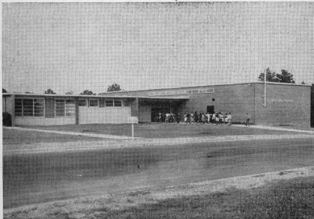
Exuberant, young people depart from the F. D. Bluford Elementary School, thus ending their second week of study in the new and modern construction here in Greensboro. Named for the late presi-
