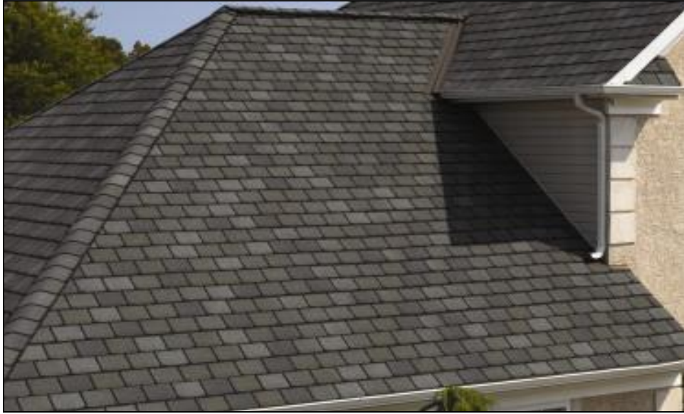
Figure 2.2 Asphalt shingles on a residential roof
