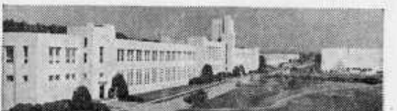
⑦ The ACOUSTICS AND VIBRATION LABORATORY was just established to intensify research and development of ships of improved detection capability, and reduced vibrations and underwater sound output. Fundamental and applied research in hydrodynamics, structural acoustics, mechanical vibrations, and signal processing are supplemented by conduct of acoustic and vibration trials, and development of acoustic and vibration instrumentation.
