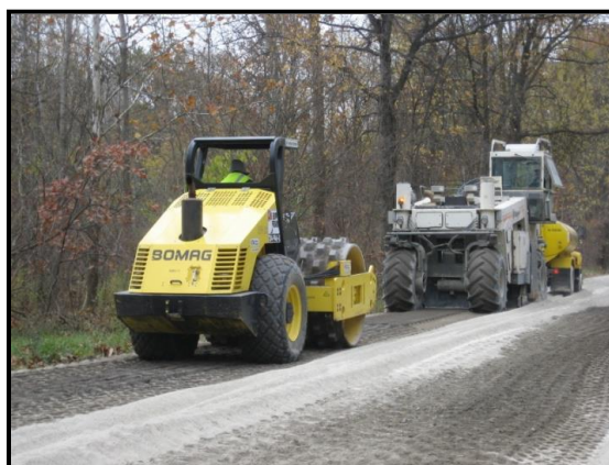
Figure 5.3. Constructing a pavement base using CKD (Courtesy of Lafarge North America).
