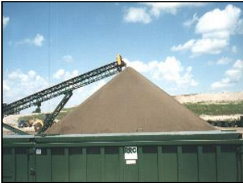
Figure 5.8. Foundry sand making plant ( www.foundryrecycling.org ).
