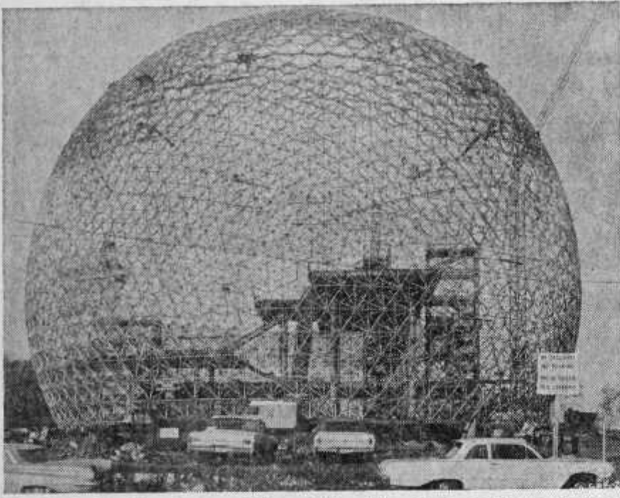
The U. S. Pavilion at Expo 67 is a $9.3 million Geodesic Dome designed by R. Buck Minister Fuller. It has a plastic skin and windows geared to the sun's progress; solo-operated cells open certain windows at certain times of the day.
