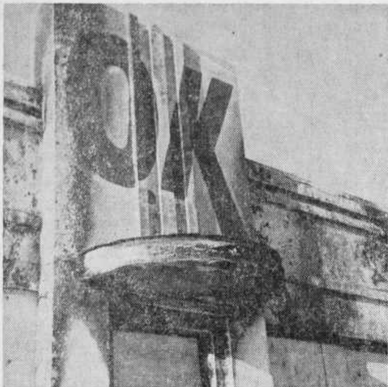
STAMP OF APPROVAL? O. K. Tire Store, Winston-Salem, was gutted by arson during recent riots. The large red O. K. ironically appears to be a stamp of approval of the riots' carnage. Photo by Larry Wrenn.
