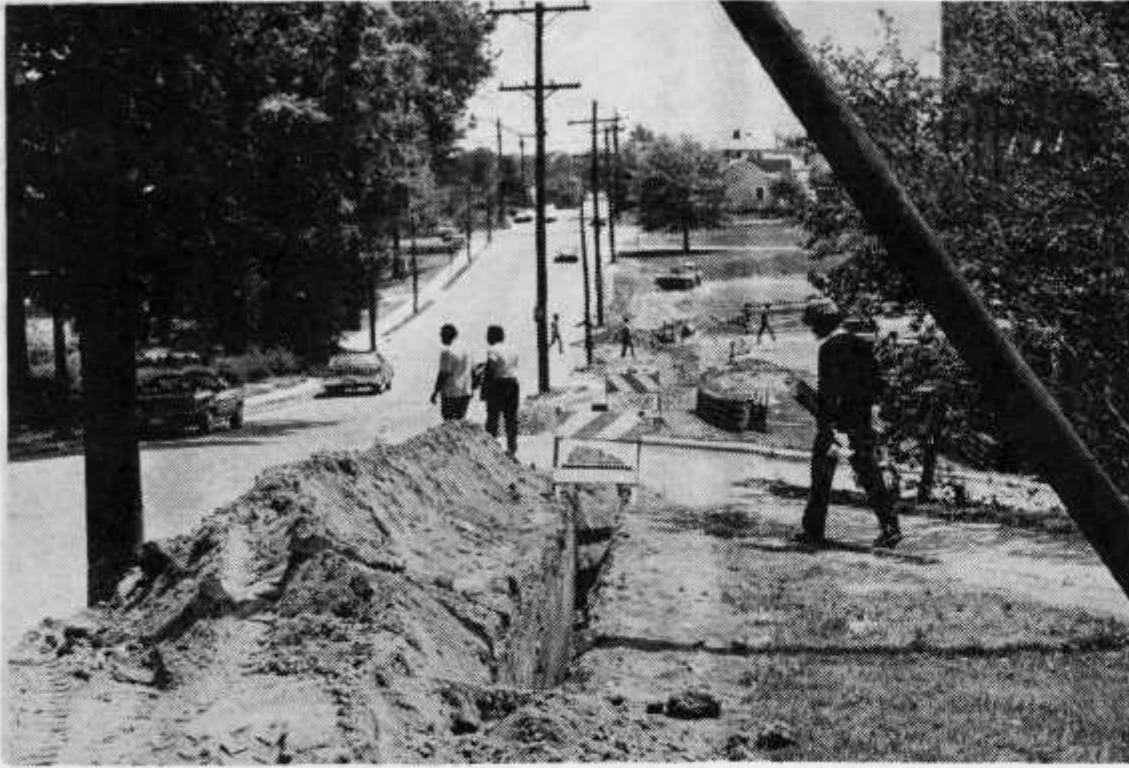
Trenches For Underground Electrical System Marr Campus As Work Continues
