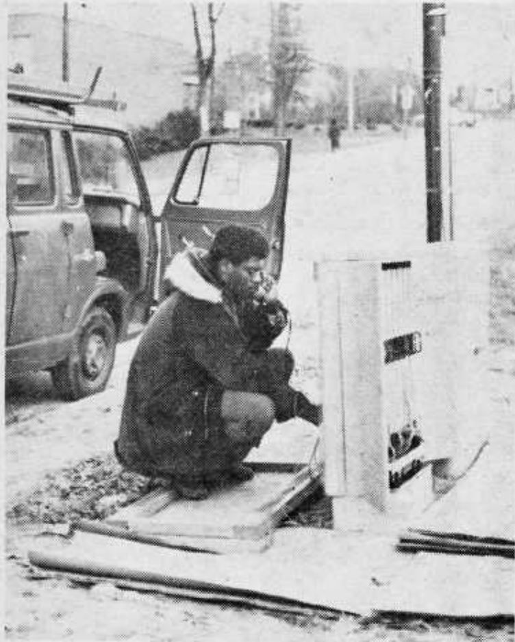
Workman Prepares Centrex Connections
