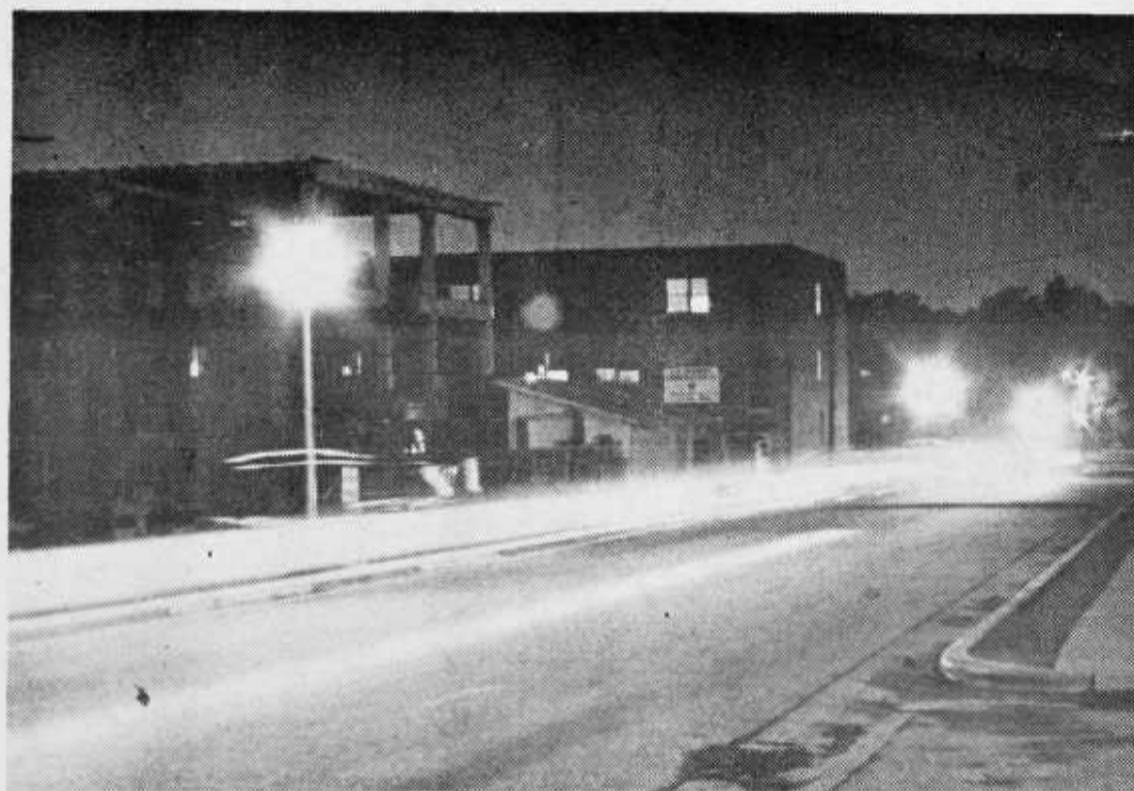
Scott Hall Construction In Night "Lite"
