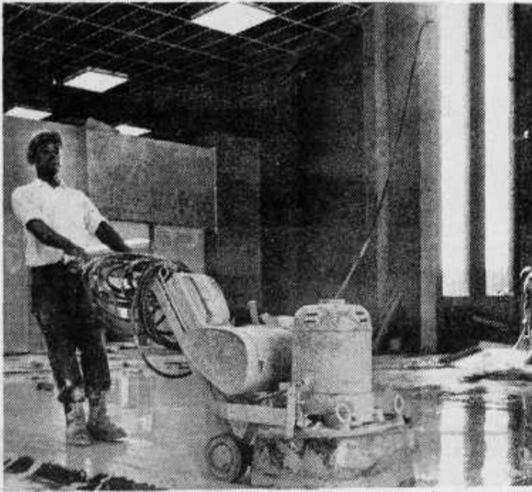
An earlier photograph of a cafeteria worker leaning into a profile as he "finishes" the floor of the new cafeteria.
