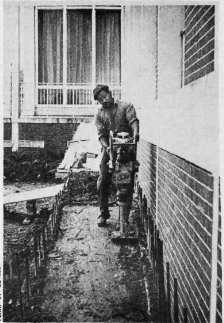
Architectural barriers are being removed.
