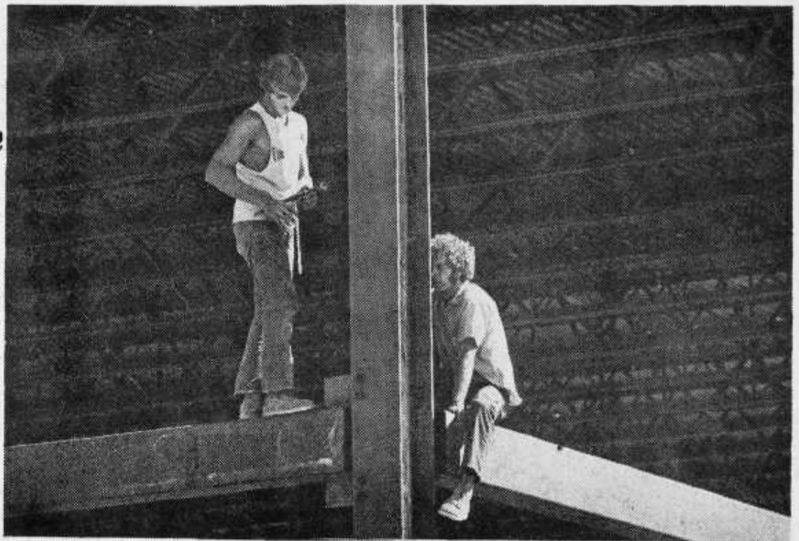
Slowly but steady, the gym is going up.
