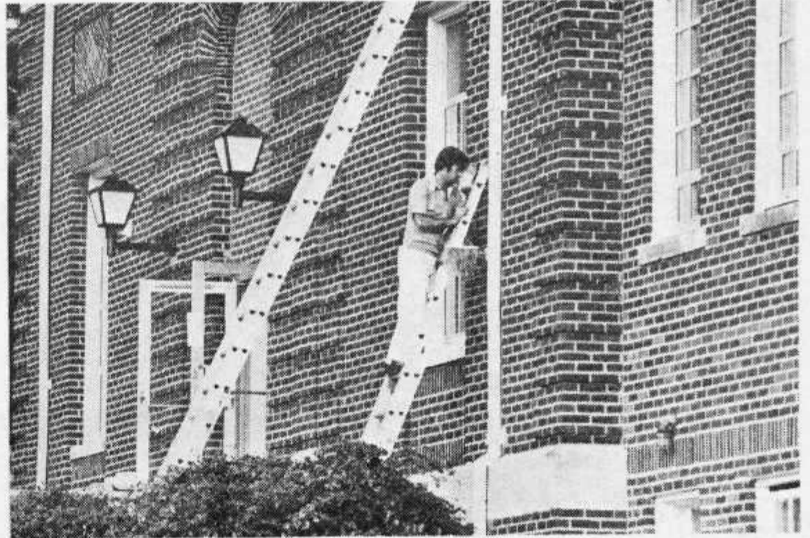
The renovation of Murphy Hall is in its final stages.
