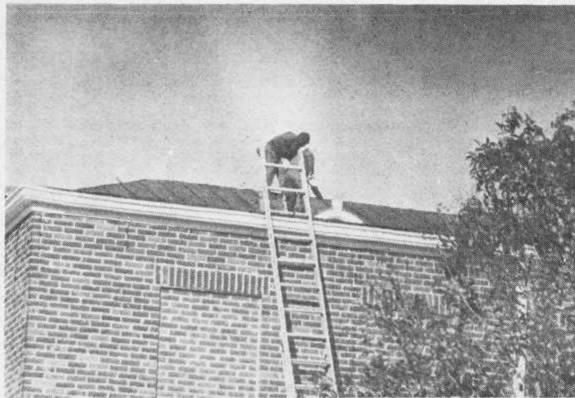
Final adjustments are made on Murphy Hall's renovation.
