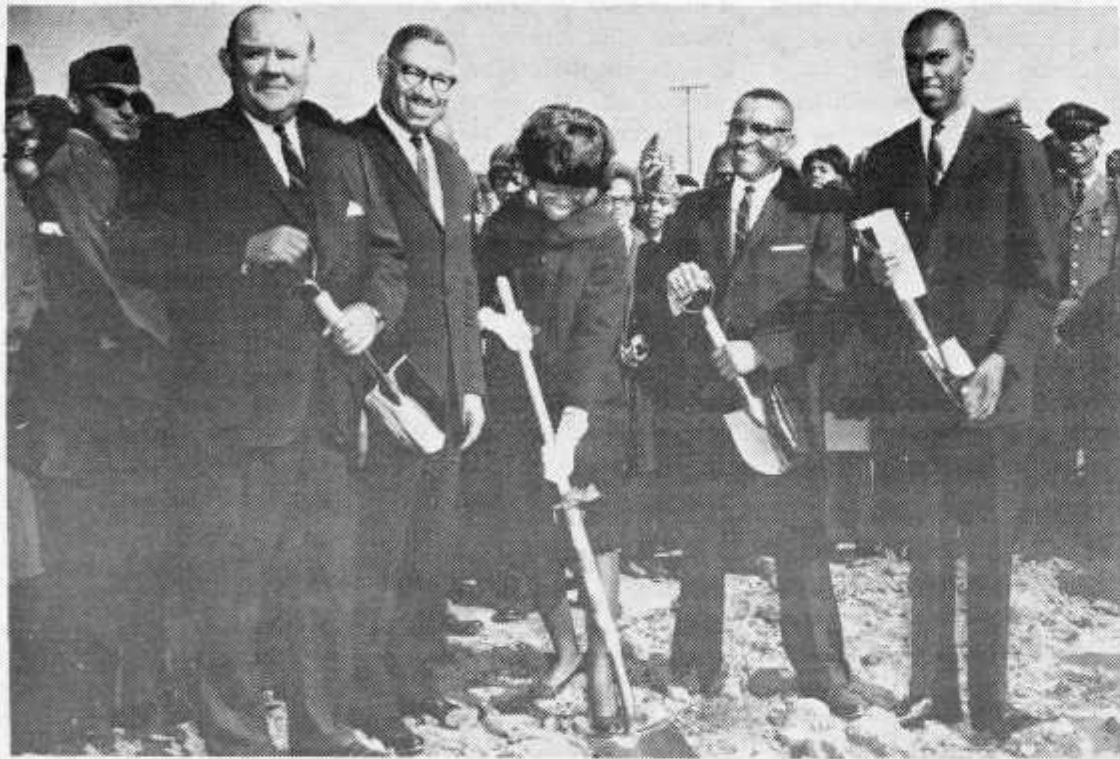
...Ground breaking of the Student Union...
