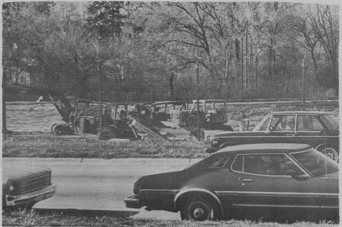
Starting work on the new stadium. (Photo by Tyson)
