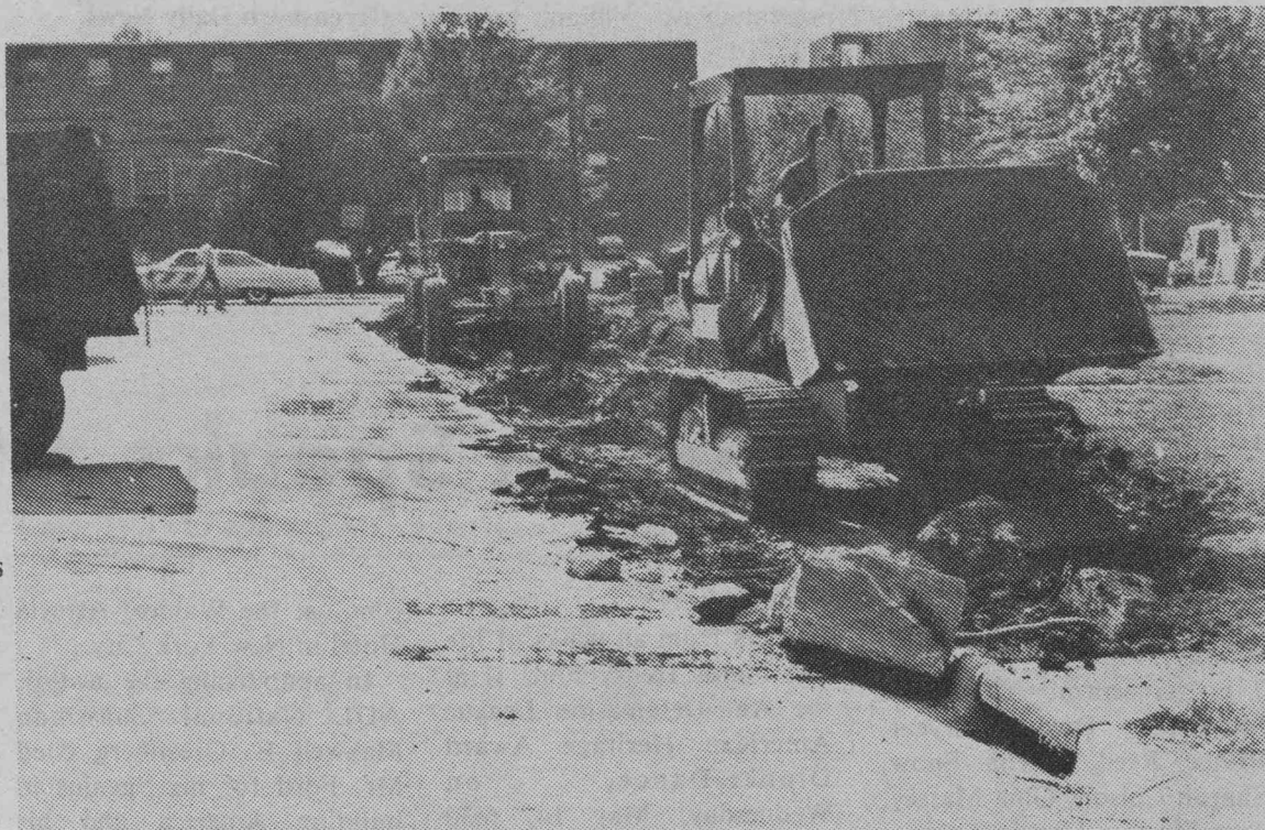
Construction is underway expanding A&T's parking facilities near Bluford Library.
