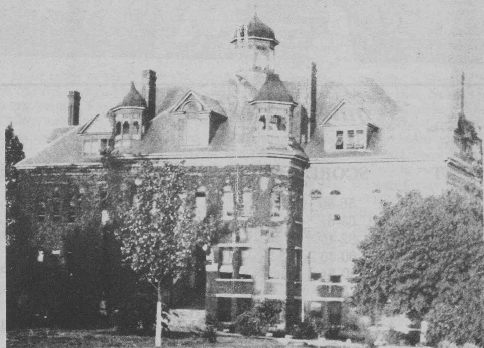
The original Dudley Building
