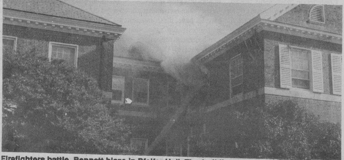
Firefighters battle Bennett blaze in Pfeifer Hall. The building was severely damaged.
